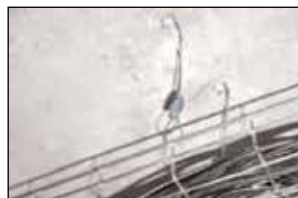
Light weight Cable Trays / Lights
