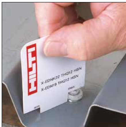
Checking the standoff of an X-EDN 19 roof deck fastening with a plastic template
