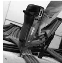
Conduits & pipes with metal or textile band
