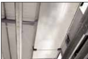
Square Air Ducts
