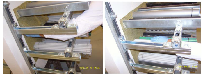
Fig. 6: Cutting and fitting mineral wool board [11]
